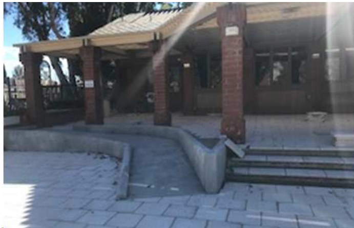
Our new ADA-compliant ramp providing access to the pool area restrooms.
